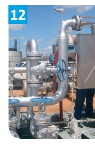
5. Fuel Oil Rheonik Coriolis mass flow meters are utilized as both transfer meters and check meters for fuel oil deliveries
